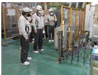
Install a guarding at the furnace (CoorsTek Nagasaki)
